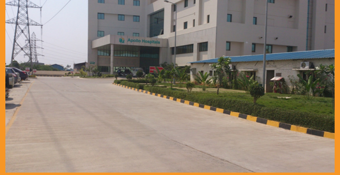
CONCRETE ROAD WORK AT APOLLO SPECIALTY HOSPITALS, VANGARAM, CHENNAI
