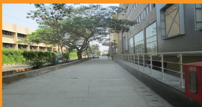
CONCRETE ROAD WORK AT FORUM VIJAYA MALL, VADAPALANI, CHENNAI
