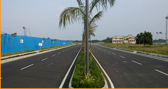
BITUMINOUS ROAD WORK AT PBEL CITY, THAYUR, KELAMPAKKAM, CHENNAI – OMR
