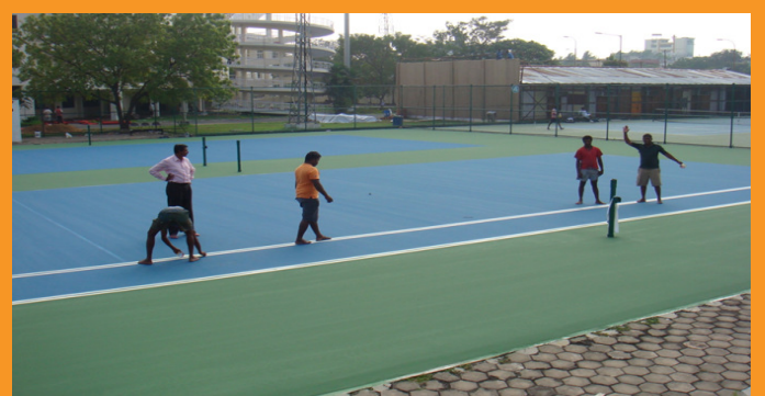
SYNTHETIC TENNIS COURT WORK AT SDAT TENNIS STADIUM, NUNGAMBAKKAM, CHENNAI
