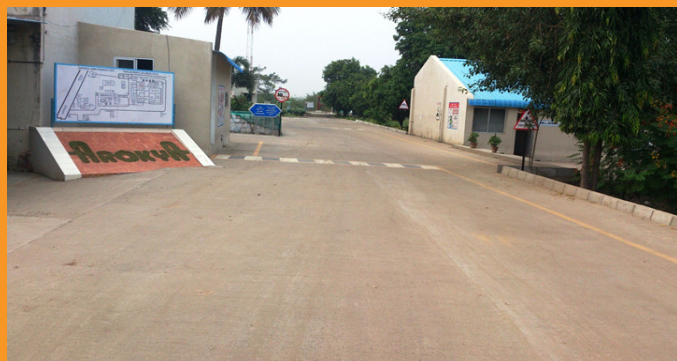
CONCRETE ROAD WORK AT HATSUN AGRO PRODUCT LIMITED, THALAIVASAL, SELAM
